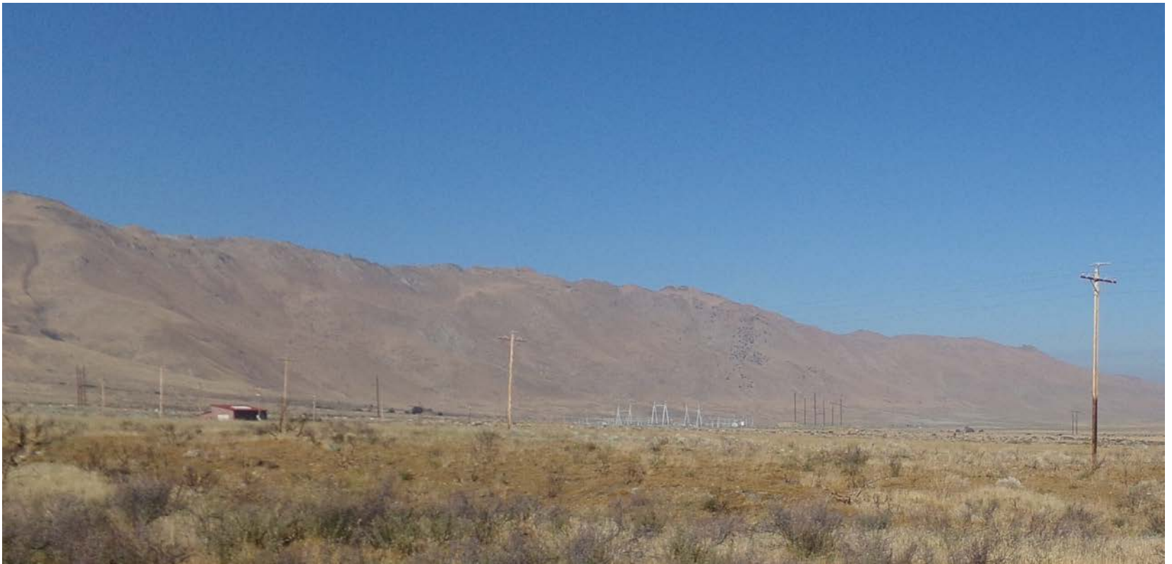
Adjacent Transmission and Fort Sage Substation
